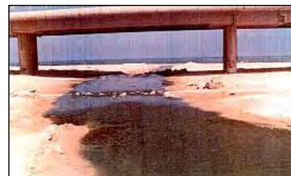
Pollution by leaching wastewater in Gaza.
